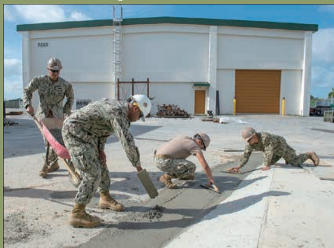
(U.S. Navy photo by Mass Communication Specialist 1st Class Stephane Belcher) ^ U.S. Navy Seabees deployed with Naval Mobile Construction Battalion (NMCB) 5 smooth concrete with magnesium floats at the ramp wing construction project for the K-Span Warehouse on board Camp Shields, Jan. 7. The Seabees deployed to Okinawa with NMCB-5 are installing a ramp wing to improve operational logistics efficiency.
