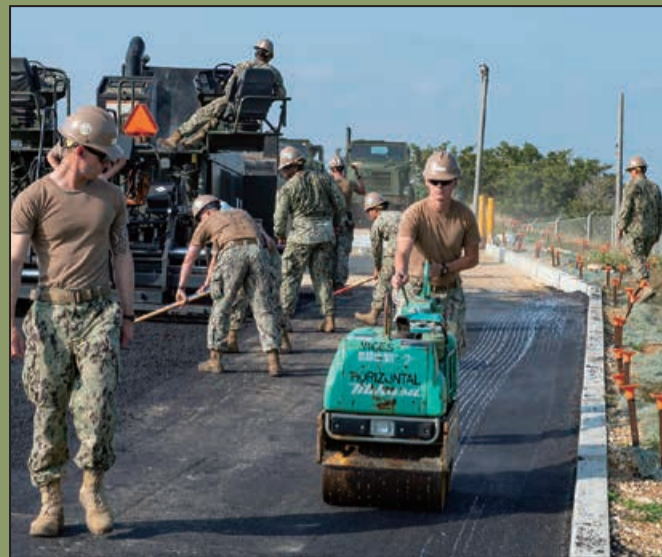
(U.S. Navy photo by Mass Communication Specialist 1st Class Stephane Belcher) ^ Builder Constructionman Brendan Lewison compacts asphalt with a walk-behind roller, while Builder 3rd Class Justin Berglund guides him on board Marine Corps Air Station Futenma, Jan. 11. U.S. Navy Seabees deployed with Naval Mobile Construction Battalion (NMCB) 5 are constructing support facilities for Marine Air Control Squadron 4's Ground/Air Task Oriented Radar System.
