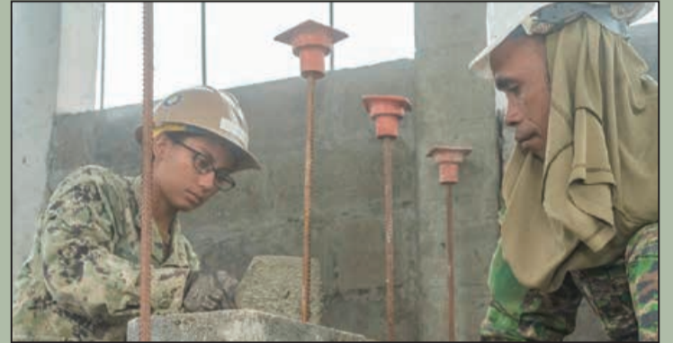
Construction Electrician 3rd Class Ana Jaramillo-Arroyo (left) assigned to Naval Mobile Construction Battalion (NMCB) 4, works with a counterpart from the Timor-Leste Defense Force to lay masonry blocks for the wall of the four-stall bathroom facility, June 3.
