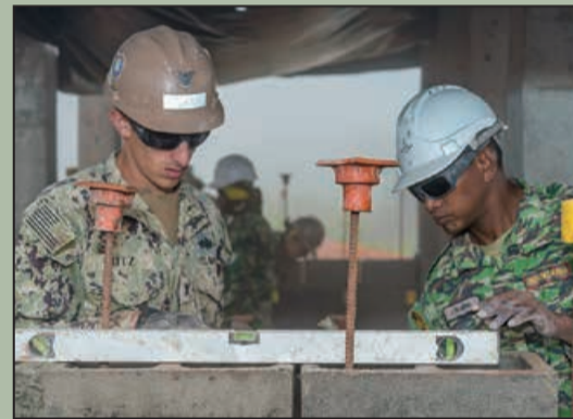
Construction Electrician 3rd Class Ana Jaramillo-Arroyo (left) assigned to Naval Mobile Construction Battalion (NMCB) 4, works with a counterpart from the Timor-Leste Defense Force to lay masonry blocks for the wall of the four-stall bathroom facility, June 3.
