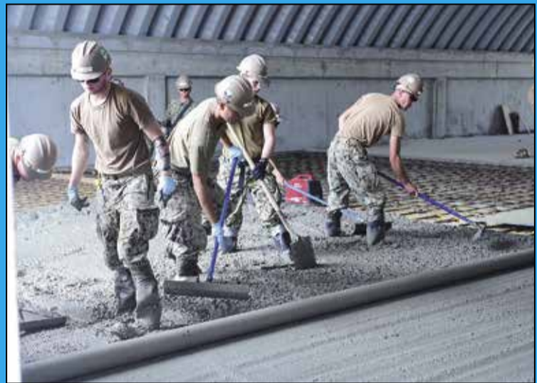
Seabees assigned to Naval Mobile Construction Battalion 3 place concrete for the construction of a k-span structure onboard Camp Shields, April 3. NMCB-3 is forward deployed throughout the Indo-Pacific region and United States ready to support major combat operations, theater security, humanitarian assistance and disaster relief operations.
