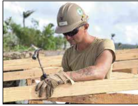
(U.S. Navy photo by Construction Electrician Constructionman Manuel Torres)
