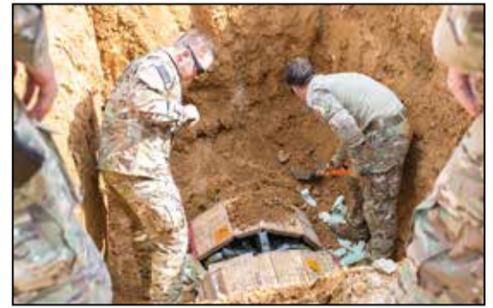
Dirtboys from the 18th Civil Engineer Squadron dig a hole as members from the 18th CES Explosive Ordnance Disposal team discuss plans for the day March 14, at Kadena Air Base. The Dirtboys work with the EOD team to ensure explosives are safely disposed of.
