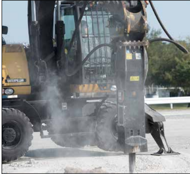
◀ Airmen from the 18th Civil Engineer Squadron train a member of the Japan Air Self-Defense Force on the correct operation of an impact hammer attached to an excavator during flightline repair training Feb. 28, at Kadena Air Base.
