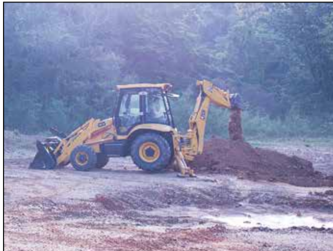
Dirtboys from the 18th Civil Engineer Squadron dig a hole as members from the 18th CES Explosive Ordnance Disposal team discuss plans for the day March 14, at Kadena Air Base. The Dirtboys work with the EOD team to ensure explosives are safely disposed of.
