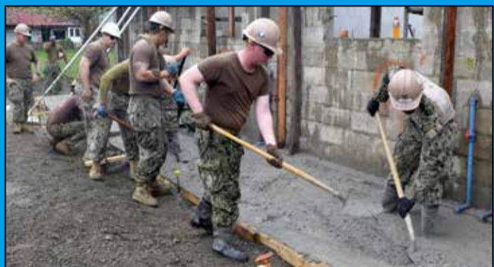
(U.S. Navy photo by Construction Electrician Constructionman Ashley Concepcion)
