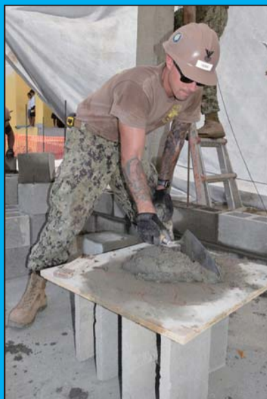
(U.S. Navy photo by Construction Electrician 3rd Class Ji Han)
